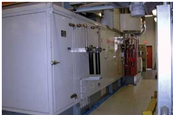
Gas turbine generator at the facility.
